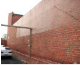
52 Edward Street Bendigo wall
