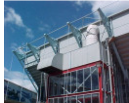
H1977 former Olympic pool
