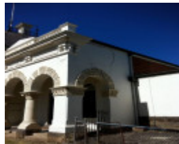
Before Photograph - Reference F3919 2014
