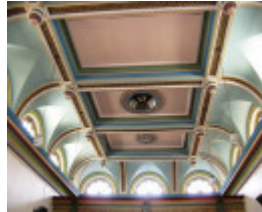
H2180 Clunes Town Hall - Hall ceiling 023
