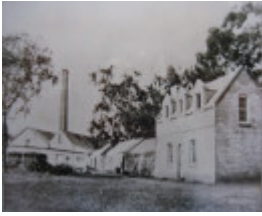
2063 Colbinabbin Homestead Former Woolscour and Associated Buildings date unknown
