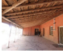
verandah of 1854 addition Sept 2015.JPG
