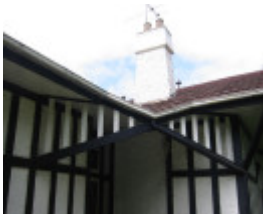
h01009 desbrowe annear house 38 the eyrie eaglemont entry eaves feb mz
