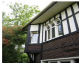
h01009 desbrowe annear house 38 the eyrie eaglemont bay window feb mz
