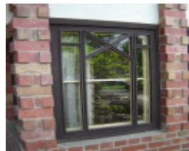
H2091 Lippincott House Glenard Dr Heidelberg Window Detail 01 Nov2005 mz
