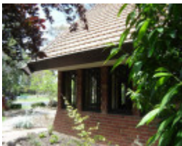
H2091 Lippincott House Glenard Dr Heidelberg Corner Window Detail Nov2005 mz
