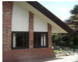
H2091 Lippincott House Glenard Dr Heidelberg Window Detail 02 Nov2005 mz
