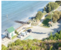
Pier boat ramp from above
