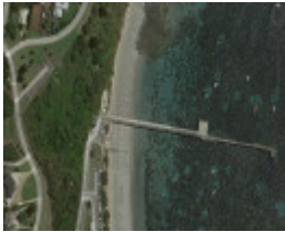
Flinders Pier from above 2018
