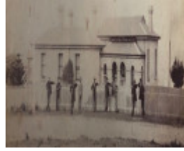
First cable station and PO
