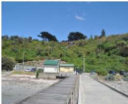
Cable landing site 2
