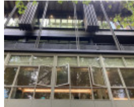
View looking upwards from Ridgway Place
