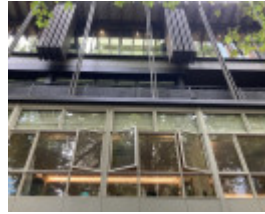
View looking upwards from Ridgway Place
