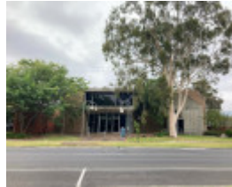
Moe Court Front of Building Feb 2022
