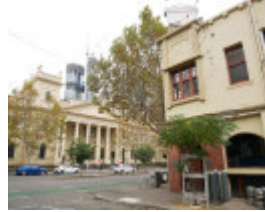
2022 view to trades hall
