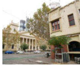
2022 view to trades hall
