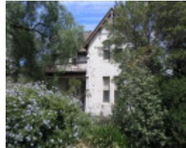
HOLY TRINITY CHURCH, VICARAGE AND HALL SOHE 2008
