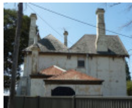
H1734 HOLY TRINITY CHURCH, VICRAGE AND HALL LHA 2015 6.JPG
