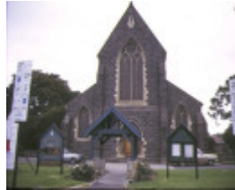
1 holy trinity church vicarage & hall nelson place williamstown church front view may1998
