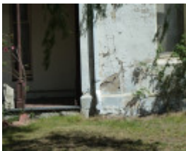
H1734 HOLY TRINITY CHURCH, VICRAGE AND HALL LHA 2015 4.JPG
