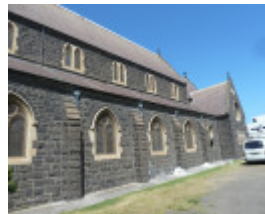
H1734 HOLY TRINITY CHURCH, VICRAGE AND HALL LHA 2015 2.JPG
