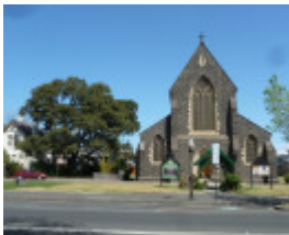
H1734 HOLY TRINITY CHURCH, VICRAGE AND HALL LHA 2015 1.JPG
