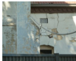
H1734 HOLY TRINITY CHURCH, VICRAGE AND HALL LHA 2015 5.JPG
