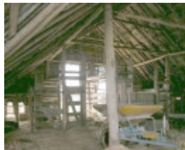
Staplegrove Meat Works Interior
