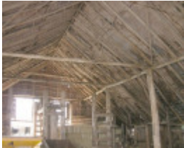
Staplegrove Meat Works Interior
