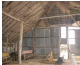
Staplegrove Meat Works Interior
