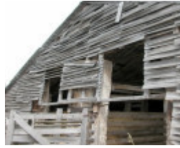
Staplegrove Meat Works Weatherboard Detail
