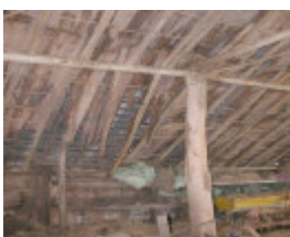
Staplegrove Meat Works Interior Framing
