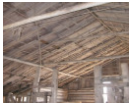
Staplegrove Meat Works Interior
