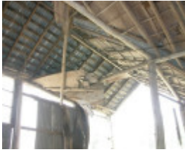
Staplegrove Meat Works Interior
