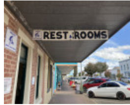
2022, Warracknabeal Ladies Rest Rooms, view south along Scott Street
