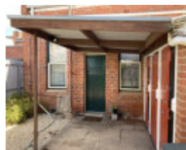
2022, Warracknabeal Ladies Rest Rooms, back door & covered area
