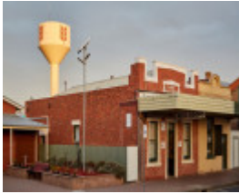
2021, Warracknabeal Ladies Rest Rooms northern elevation
