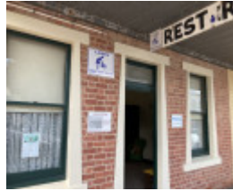
2022, Warracknabeal Ladies Rest Rooms, western elevation
