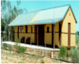
August 2022 Former Irymple Railway Station Building
