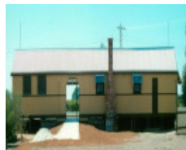
2022, Station building at Red Cliffs after 2001 restoration
