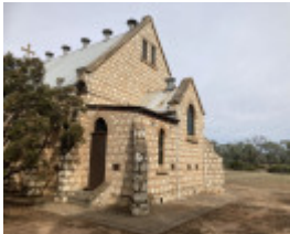
Northern elevation of church (rear entrance)
