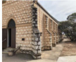
Southeast elevation of church
