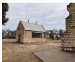
April 2023, Eastern elevation of school building
