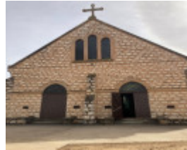
Southern elevation of church (front entrance)
