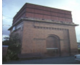
Elmore Railway Station Water Tower (1984)
