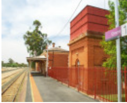
Elmore Railway Station and Water Tower
