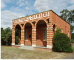
Former Huntly Shire Council Chambers
