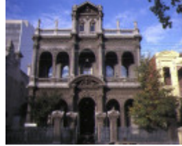
1 Benvuta Drummond Street Carlton front view
