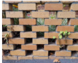
2024 - detail - hit and miss cream brick fence
