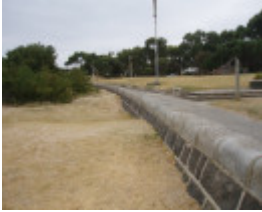
21305 Bluestone retaining wall
