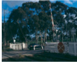
Brunswick Road Level Crossing Gates
