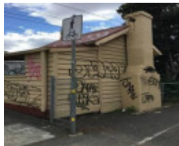
Brunswick Street Gatekeepers cabin.jpg
