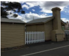
Park St gatekeepers cabin.jpg
