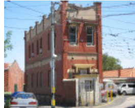
TRAM DEPOT SOHE 2008
