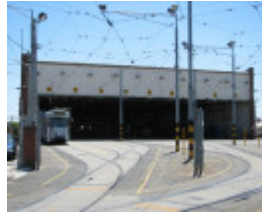
TRAM DEPOT SOHE 2008
