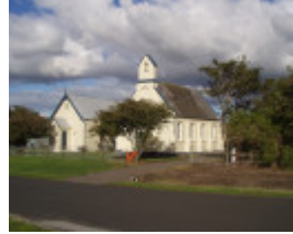
Church & Hall, Church Road Bellarine - Photo 1
