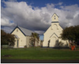
Church & Hall, Church Road Bellarine - Photo 1
