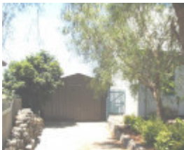
27 Harding Street, Portarlinton - Exterior - Garage
