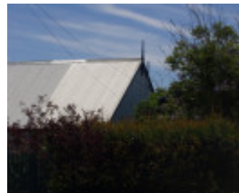
27 Harding Street, Portarlinton - Exterior - Roof
