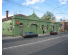
Northcote Tramways Building Thornbury Oct 2007 m/z High Street Elevation
