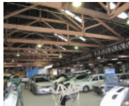
Northcote Tramways Building Thornbury May 2009 m/z Engine House Interior 01
