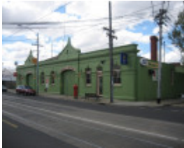
Northcote Tramways Building Thornbury Oct 2007 m/z Front Elevation 01
