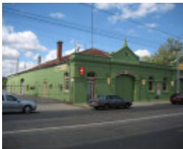
Northcote Tramways Building Thornbury Oct 2007 m/z Front 7 North Elevations
