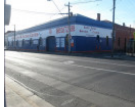
Brunswick cable tram engine house
