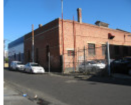
Brunswick cable tram engine house - substation
