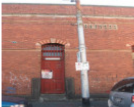
Brunswick cable tram engine house substation entrance
