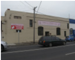
Brunswick cable tram engine house 261-63 Brunswick Road
