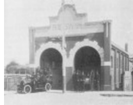
Geelong West Fire Station c.1922_resize.jpg
