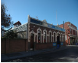
Office - 77-79 Lt Malop Street, Geelong
