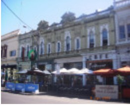
'Salisbury Buildings', Hobsons Bay Heritage Study 2006
