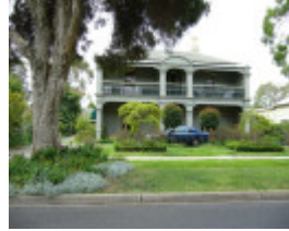
House and Pepper Trees at 54 Osborne Street, Hobsons Bay Heritage Study 2006
