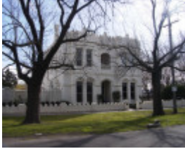
Tudor House at 52-54 Pasco Street WILLIAMSTOWN, Hobsons Bay Heritage Study 2006
