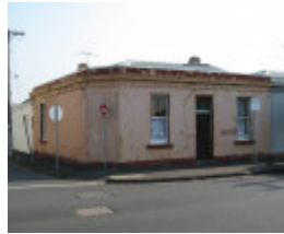
Shops (former) and Residences at 46-48 Stevedore Street WILLIAMSTOWN, Hobsons Bay Heritage Study 2006 - No 48
