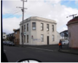
Napier Hotel (former), Hobsons Bay Heritage Study 2006
