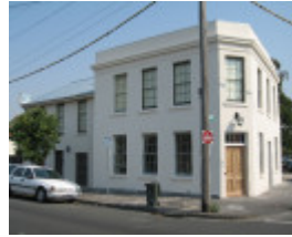
Napier Hotel (former), Hobsons Bay Heritage Study 2006
