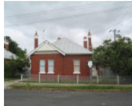
Police Station, Sergeant and Watch house Keeper Quarters (former), Hobsons Bay Heritage Study 2006 - No. 8
