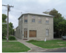
Bridge Hotel (former), Hobsons Bay Heritage Study 2006
