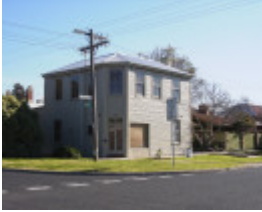
Bridge Hotel (former), Hobsons Bay Heritage Study 2006
