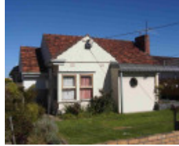
Solomit or Straw House Heritage Precinct ALTONA, Hobsons Bay Heritage Study 2006 - 173 Maidstone Street
