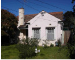
Solomit or Straw House Heritage Precinct ALTONA, Hobsons Bay Heritage Study 2006 - 169 Maidstone Street
