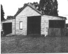
22597 Shed - 20 Monckton Road, Templestowe
