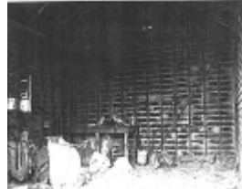
22597 Shed - 20 Monckton Road, Templestowe
