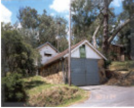
22648 Warrandyte Fire Station (former) - Mitchell Avenue, Warrandyte
