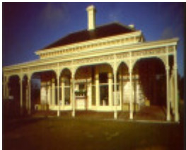
h01899 the anchorage sorrento nepean hwy
