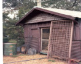
22667 Blacksmiths Building - Tills Drive, Warrandyte (2)
