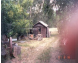
22667 Blacksmiths Building - Tills Drive, Warrandyte (1)
