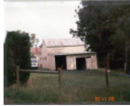
22676 Shed - 245 Tindals Road, Warrandyte (B)
