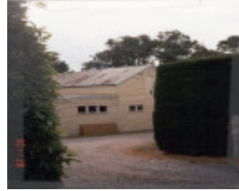
22676 Shed - 245 Tindals Road, Warrandyte (A)
