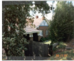
22709 Police Station (former) - 65 Yarra Street, Warrandyte
