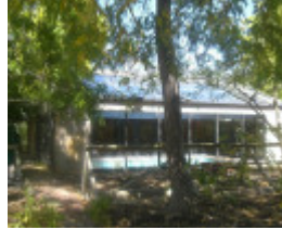
22724 House - 138-140 Brysons Road, Warrandyte South (3)
