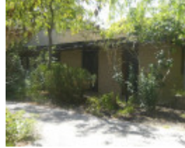
22724 House - 138-140 Brysons Road, Warrandyte South (2)
