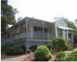
22727 House - 101-103 Brushy Park Road, Wonga Park (1)
