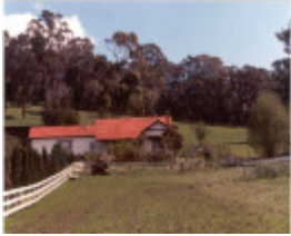
22728 House - 81 Brushy Park Road, Wonga Park
