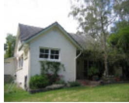
22731 House (rear) - 9 Cecil Street, Wonga Park
