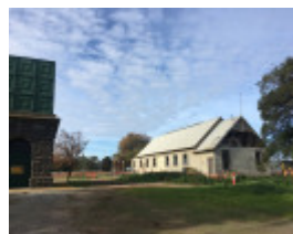
Cocoroc farm hall and Water Tank - June 2020
