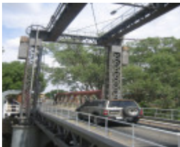
Swan Hill Bridge_Swan Hill_Feb 2008_mz_Lift Span Detail
