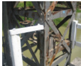
Swan Hill Bridge_Swan Hill_Feb 2008_mz_Winch
