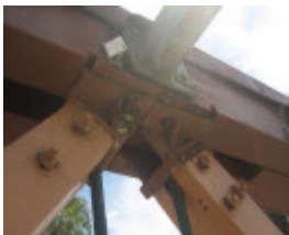
Swan Hill Bridge_Swan Hill_Feb 2008_mz_Truss Connector Detail
