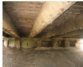
Swan Hill Bridge_Swan Hill_Feb 2008_mz_Round Timber Girders
