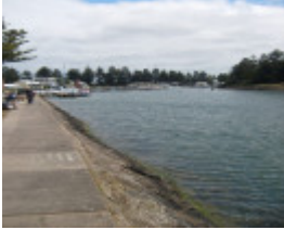
PROV H2213 Moyne River Training Walls 4
